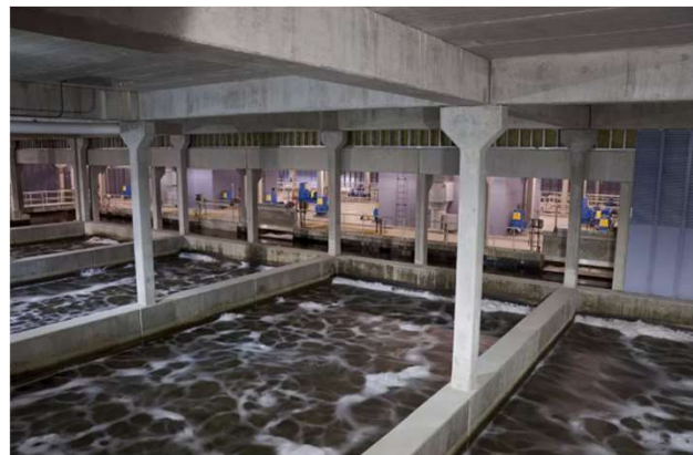
Top view of typical Veolia BAF cell
