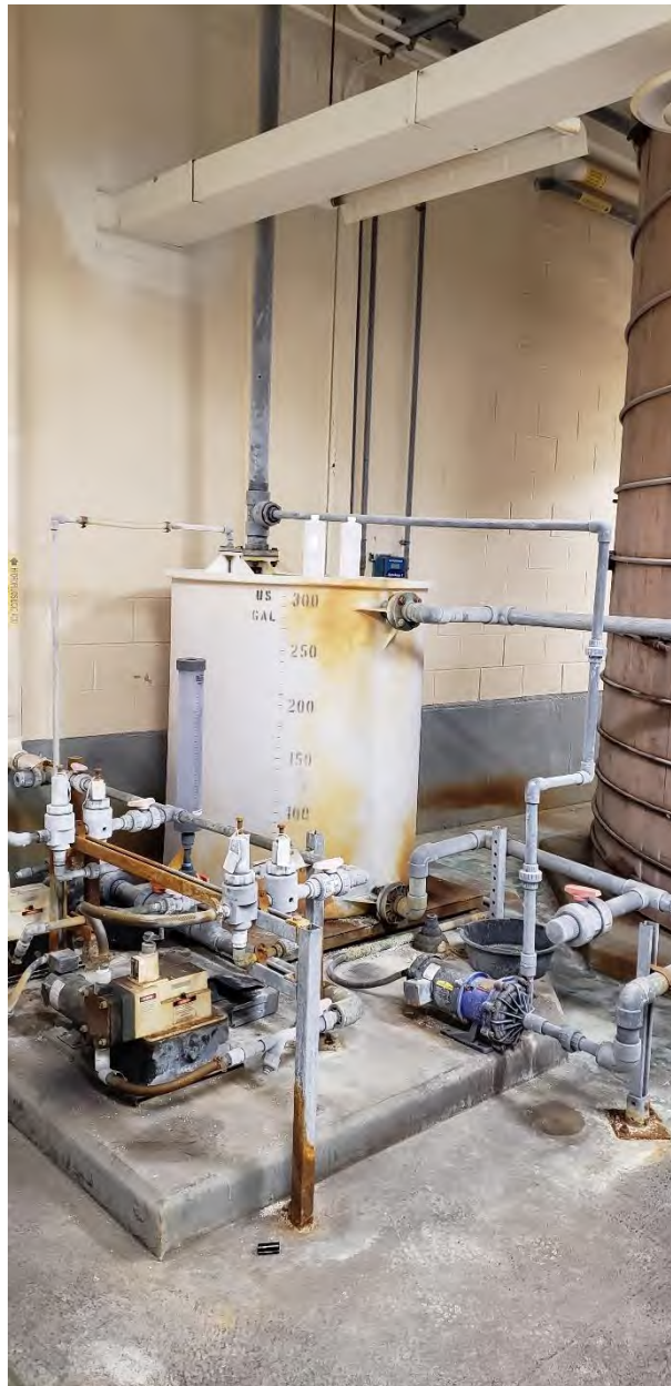
WTP-6.4 - Fluoride System Upgrades – existing chemical day tank and injection equipment in poor condition.
