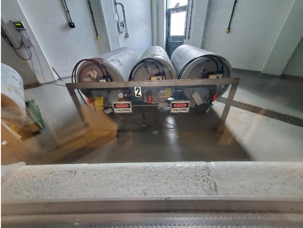
WTP-6.1 - Chlorine System Upgrades – existing, aged storage tanks
