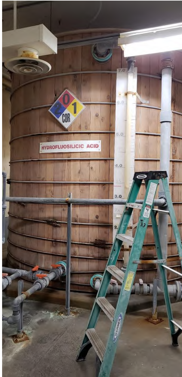
WTP-6.4 - Fluoride System Upgrades – existing chemical storage tanks with liner in need of replacement.
