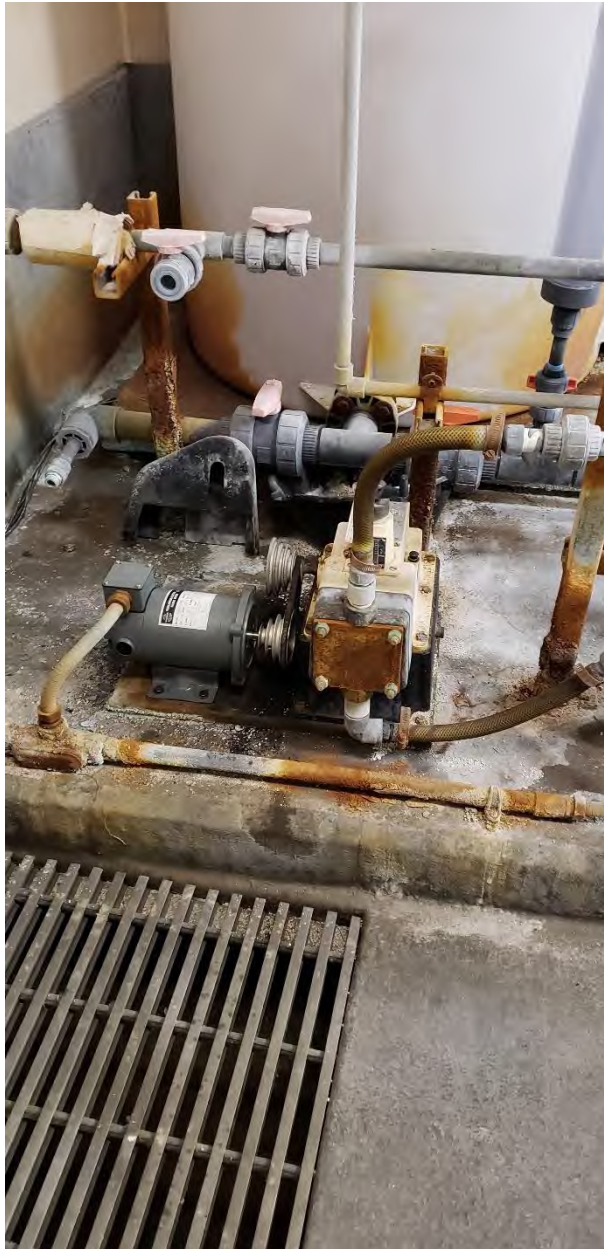
WTP-6.4 - Fluoride System Upgrades – close up view of equipment in need of replacement.
