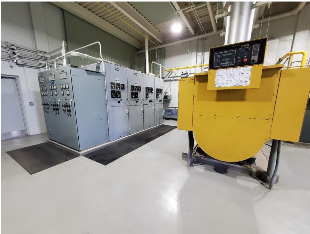
WTP-6.2 - Emergency Generator – existing, aged generator and control center
