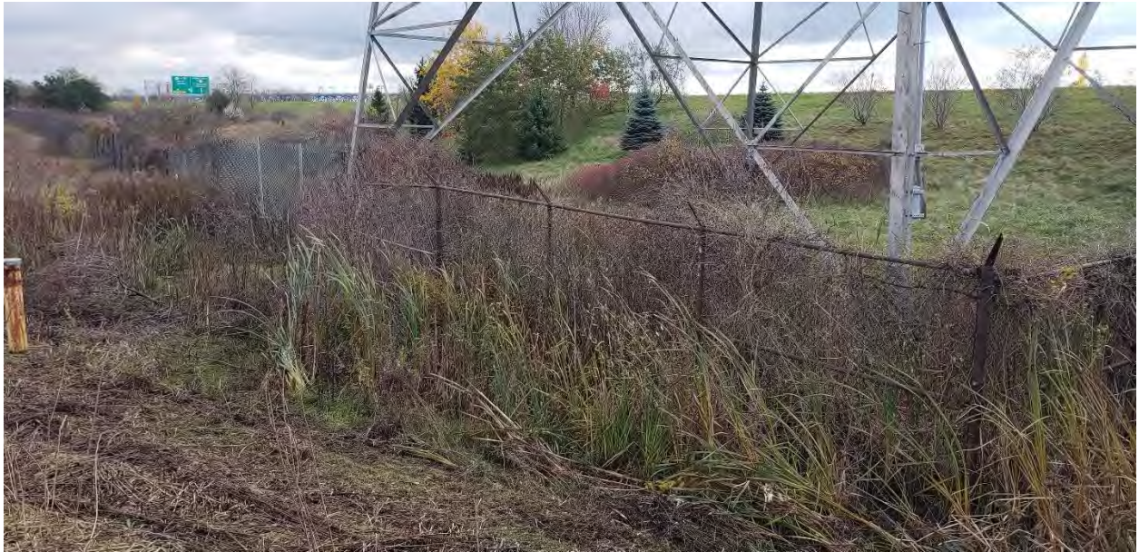
WTP-2.2 - Security Upgrades – existing chain link fence in poor condition. Located along main highway.
