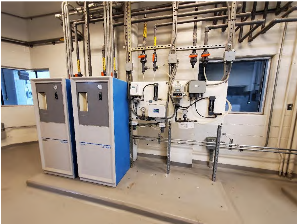
WTP-6.1 - Chlorine System Upgrades – existing, aged injection equipment
