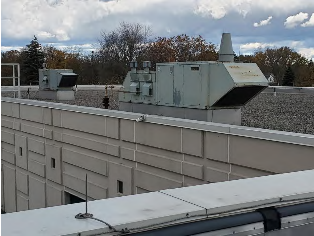
WTP-6.3 - HVAC Upgrades – existing, aged rooftop units
