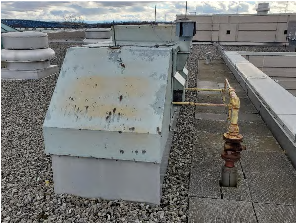
WTP-6.3 - HVAC Upgrades – existing, aged rooftop units
