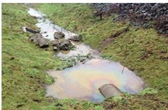
In some instances, companies and individuals have waste pipes tapped into stormwater pipes. In other cases, individuals use the storm drain inlets to dispose of various types of waste. Disposal of anything other than stormwater in storm sewers is illegal.
