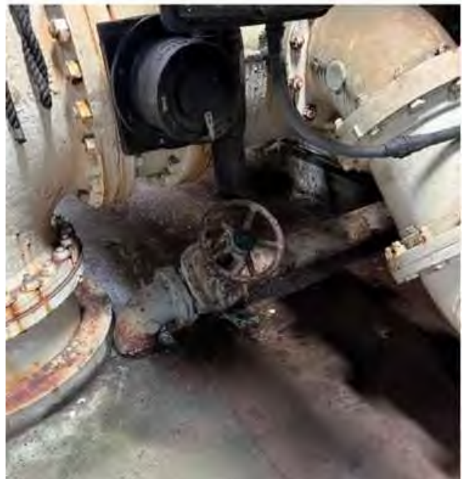
Existing mud valve with accessibility to replace.
