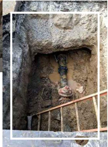
The cleaning of the watermain, mechanically removes the tuberculated build up iron oxide while the relining process reestablishes the cement lining within the watermain. The cleaning and relining of the pipe rejuvenates and extends its service life while improving service pressure and volume.
