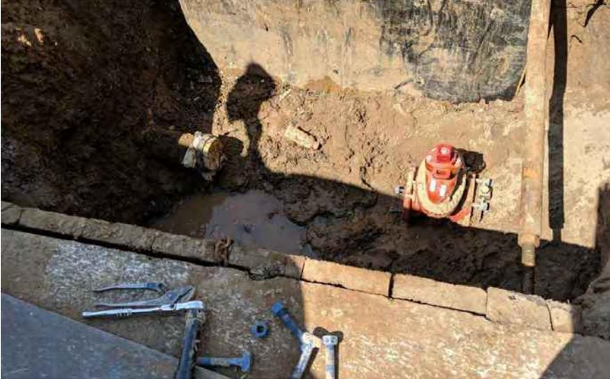
The cleaning of the watermain, mechanically removes the tuberculated build up iron oxide while the relining process reestablishes the cement lining within the watermain.
