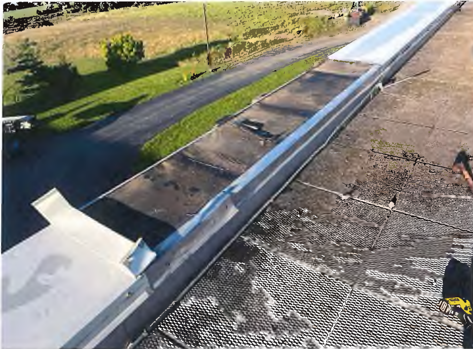
Overview of flashing after coping was removed.
