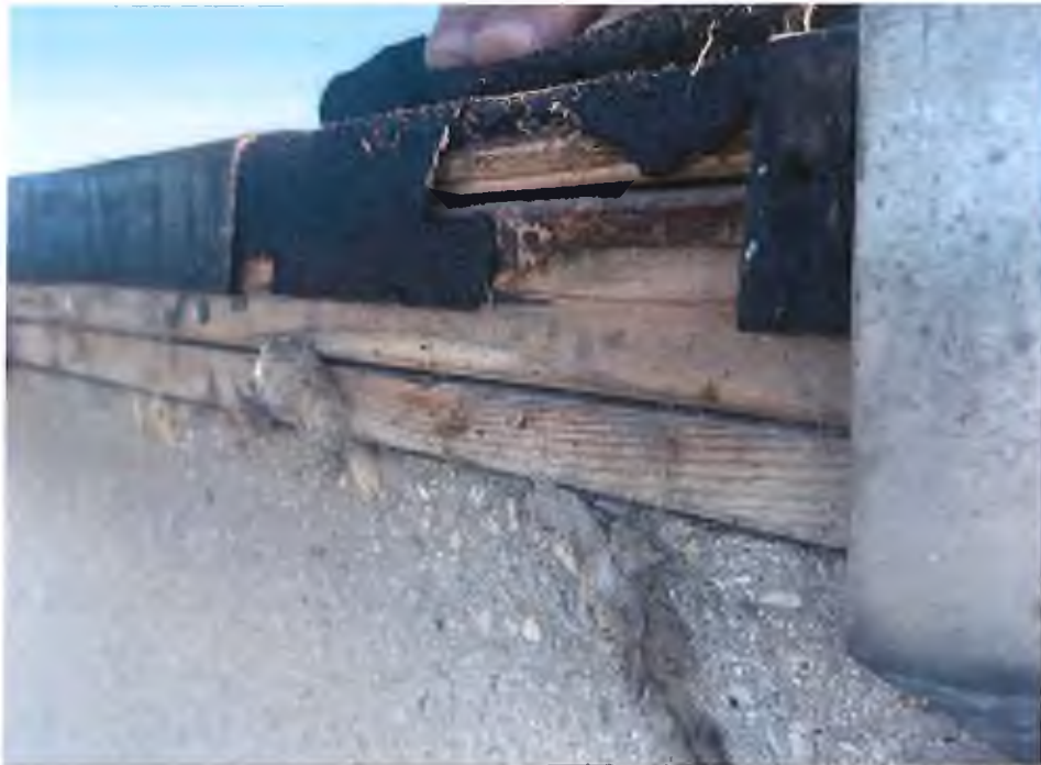
View of exterior edge of flashing/blocking. Existing did not properly cover wood blocking onto stone.
