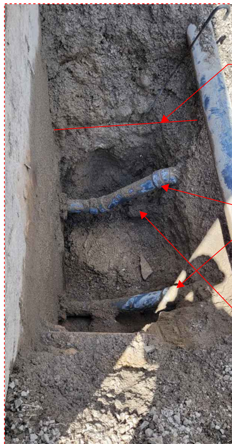
PHOTO 3 - LOOKING NORTH ALONG FRONT OF SLUDGE BUILDING WHERE THE 2 PVC SLUDGE LINE REPLACEMENTS WERE INSTALLED IN RECENT YEARS. CONCRETE WAS REMOVED AT FACE OF BUILDING TO ALLOW THESE PVC LINES TO BE INSTALLED.
