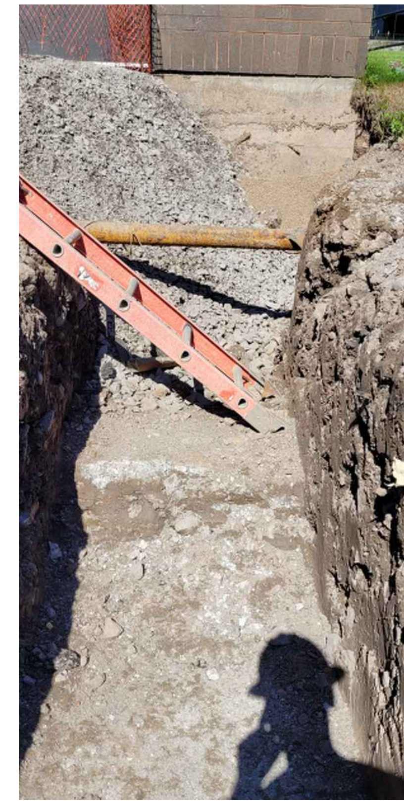
PHOTO 1 - LOOKING WEST TOWARDS SLUDGE THICKENER BUILDING. TOP OF CONCRETE ENCASEMENT IS ABOUT 2 FT THICK OVER THE SLUDGE LINES.
