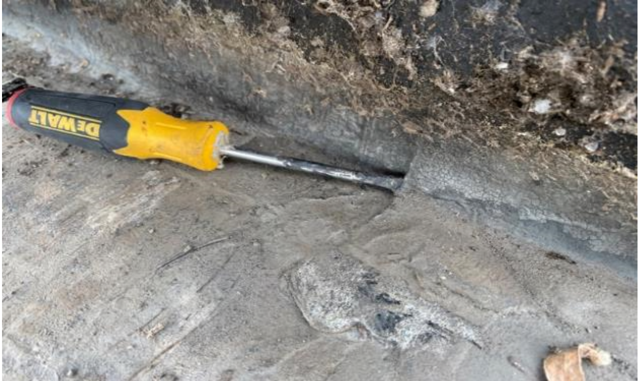
The repair team located one suspect concern in the base flashing membrane.
