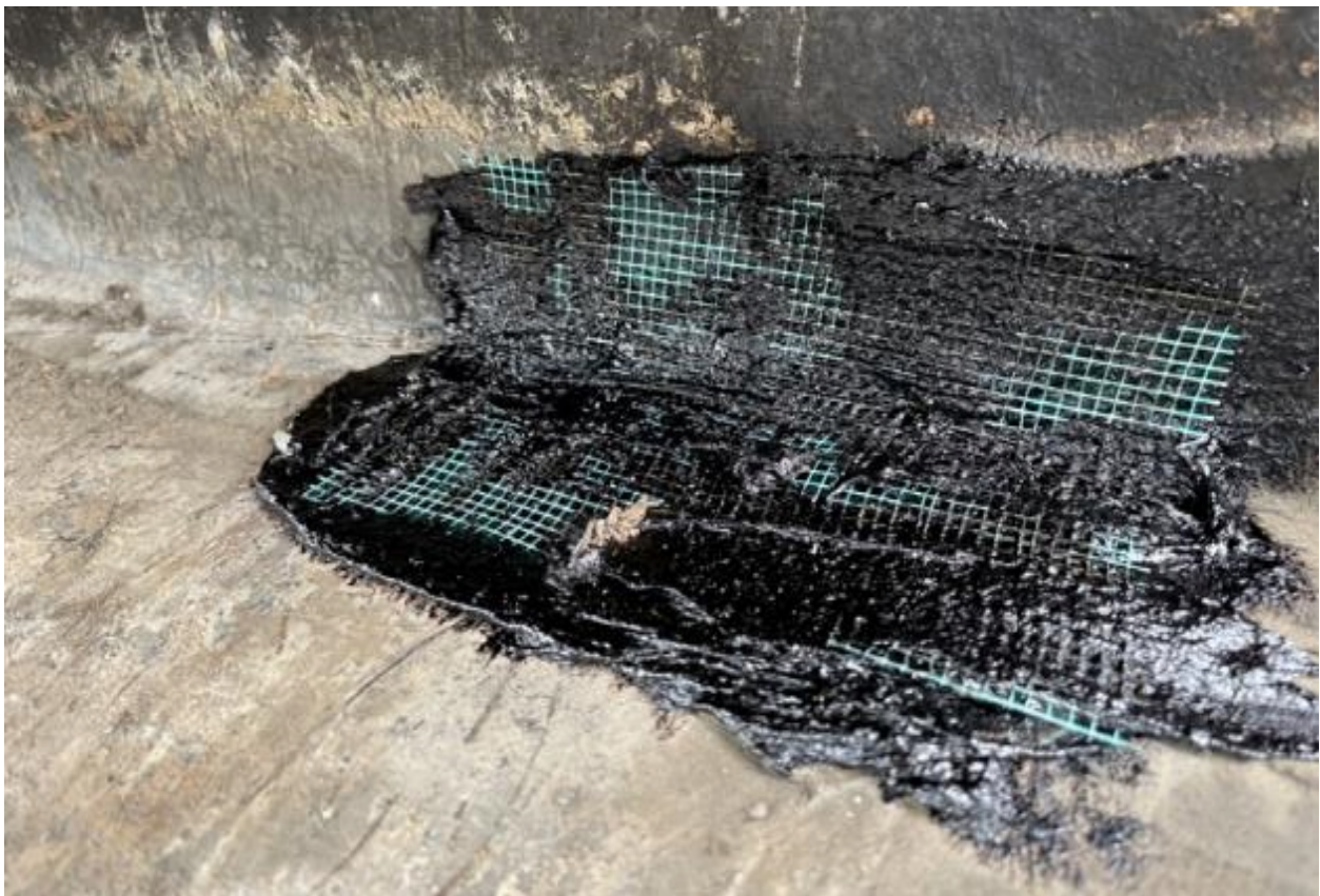
The base flashing was re-sealed with compatible materials.
