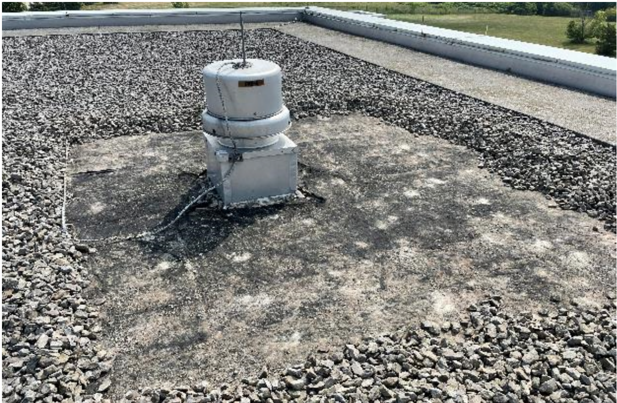
The tech rep cleared away the heavy stone ballast.
