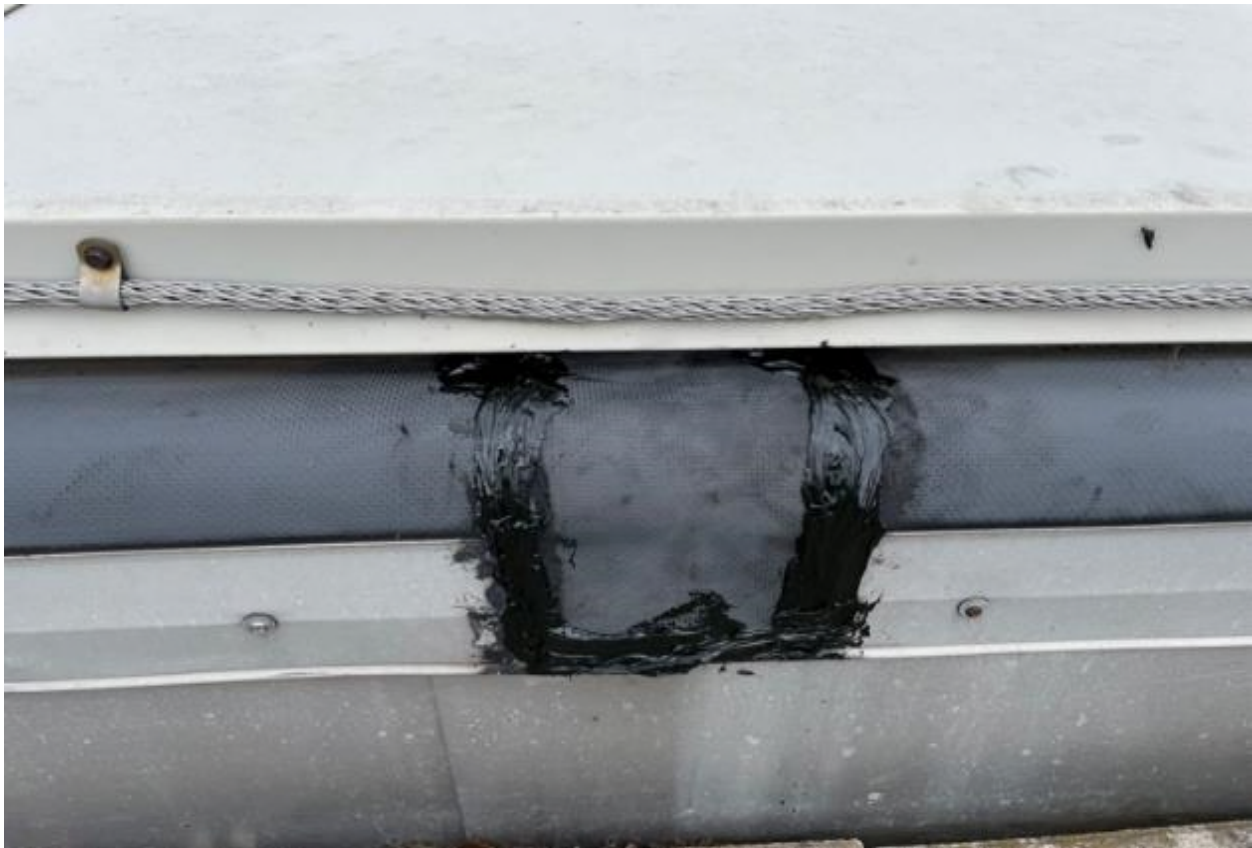
The repair team re-sealed this joint cover while on site.
