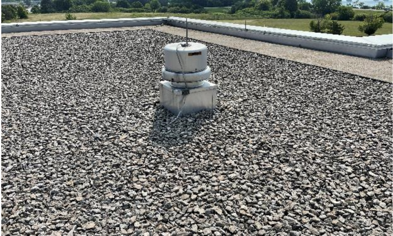
This exhaust unit is located directly above the reported “roof leak”.
