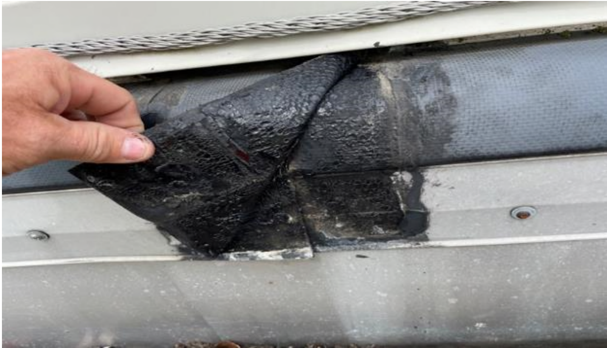
The loose membrane may be allowing some water entry.
