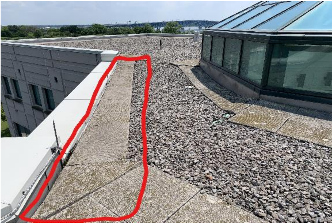
Base flashings at the perimeter edge above the building entrance-atrium are in need of inspection and possible repair.
