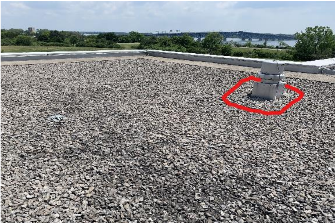
Base flashings at the fan curb above the conference room are in need of inspection and possible repair.
