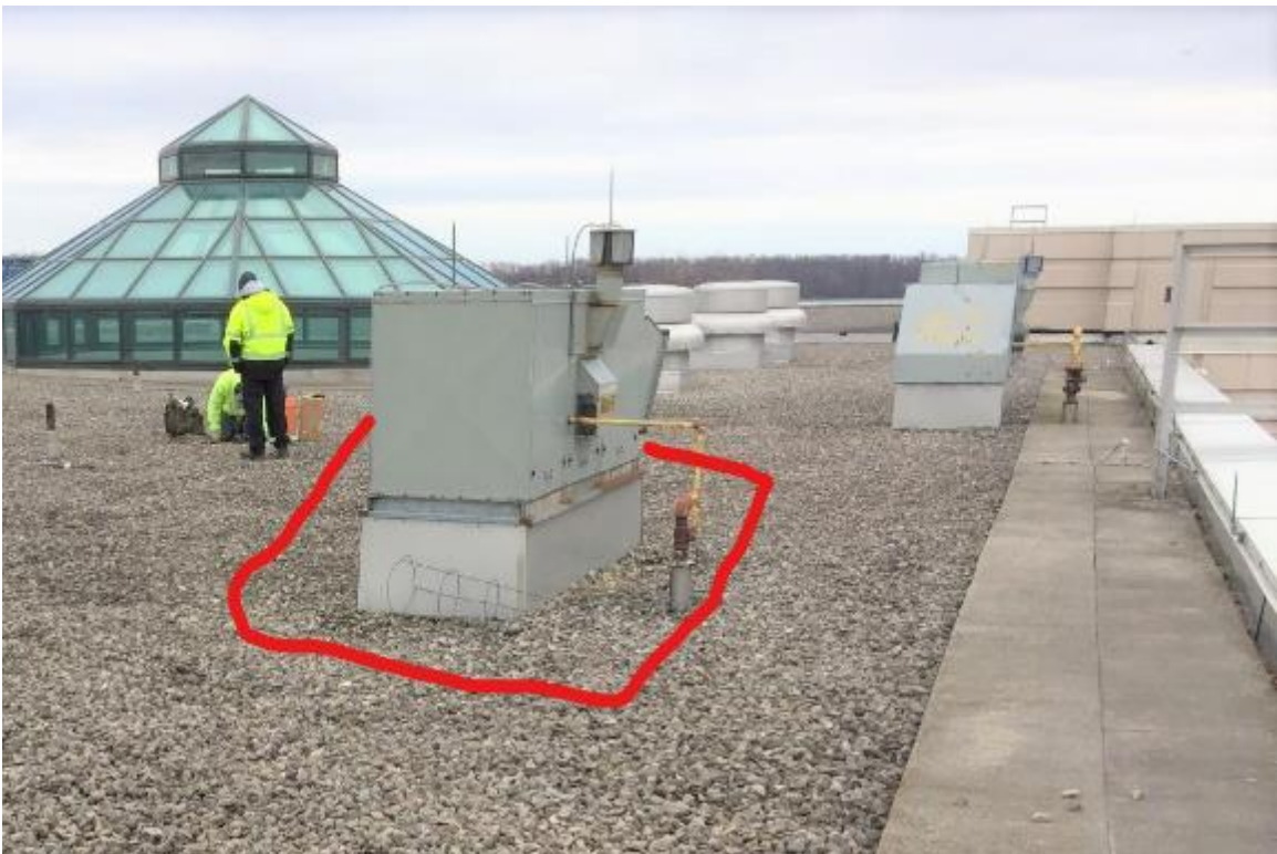
Base flashings at the large Roof Top Unit curb above the garage door are in need of inspection and possible repair.
