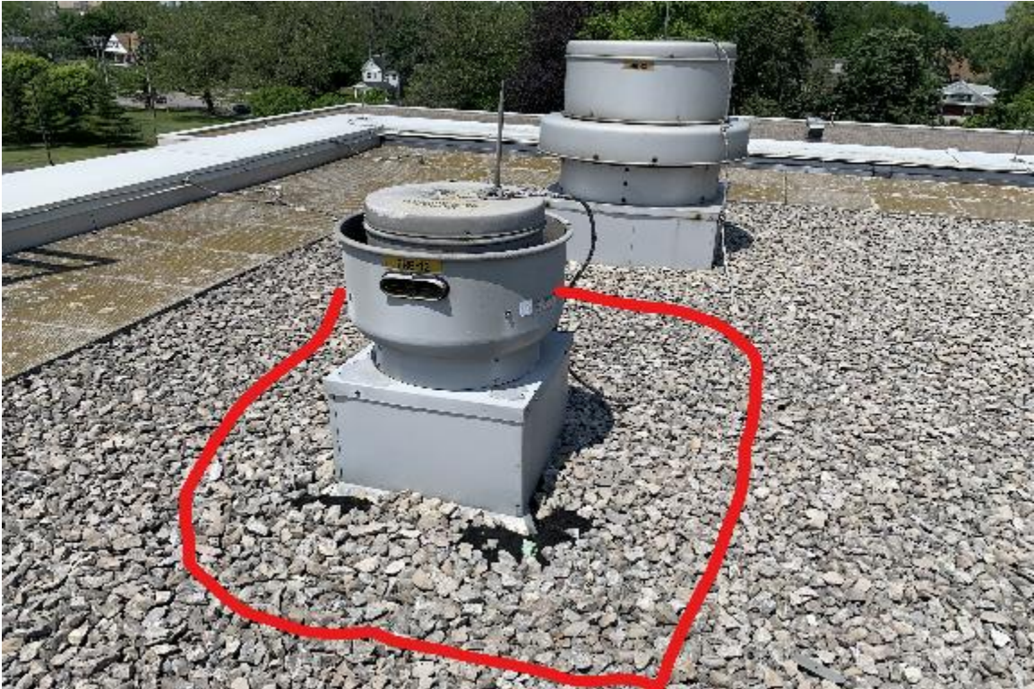
Base flashings at the fan curb above the process area are in need of inspection and possible repair.
