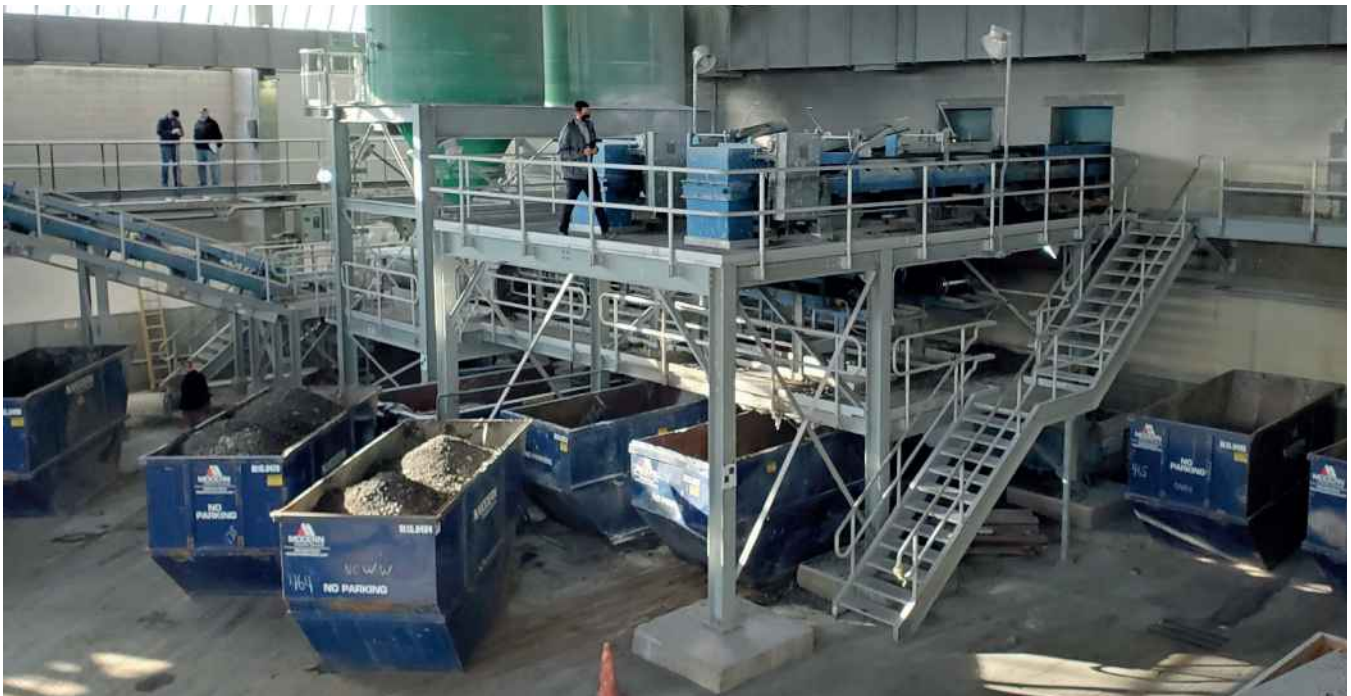
Figure 1-2 Lime Stabilization System
