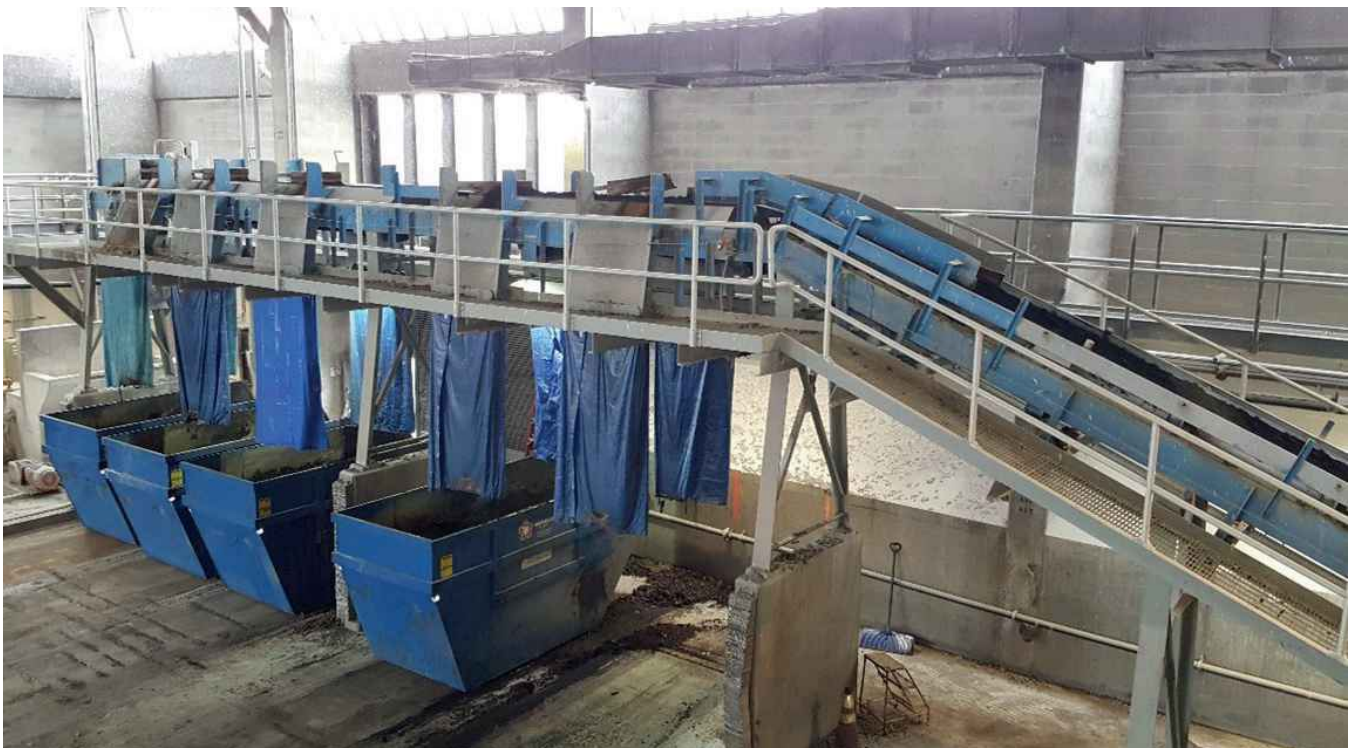
Figure 1-1 Sludge Lugger Box Loading Conveyor
