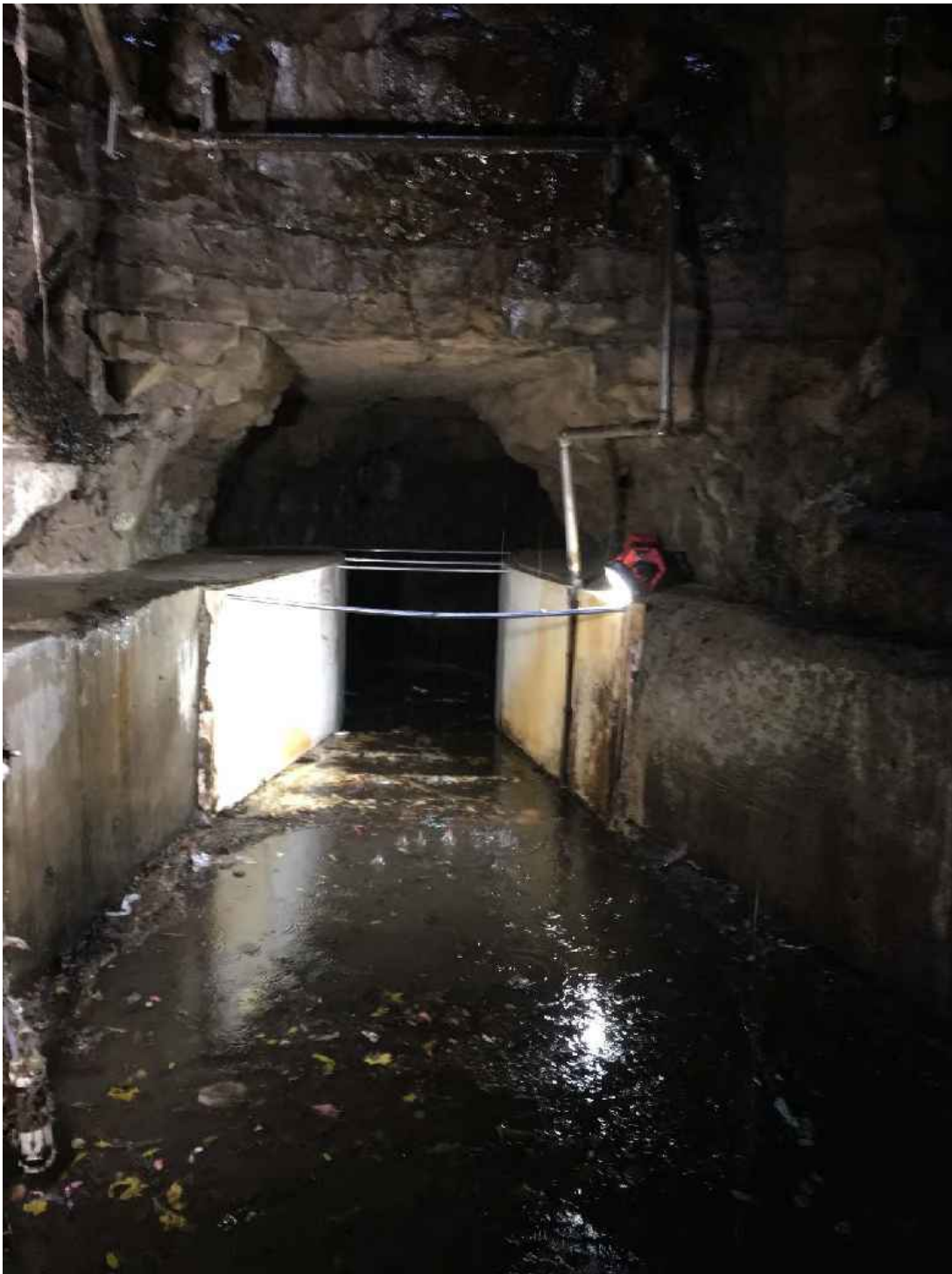
Parshall Flume (facing west, in the direction of flow)
