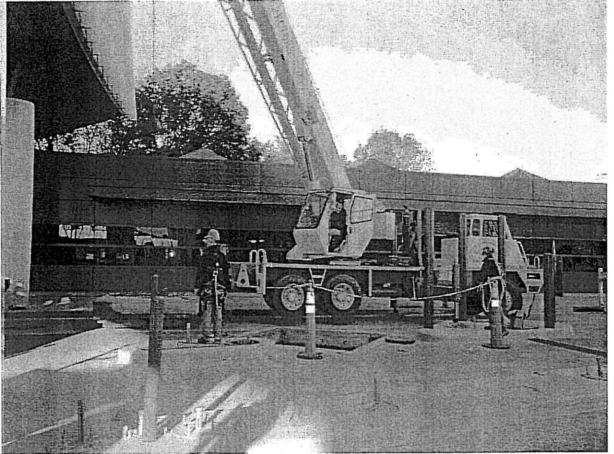
Photo 2 : Removing Falls Street Tunnel Drop Shaft Zero Vault Cover
