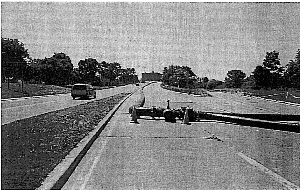
Photo 8 : Contract 52 Bypass Pipeline
